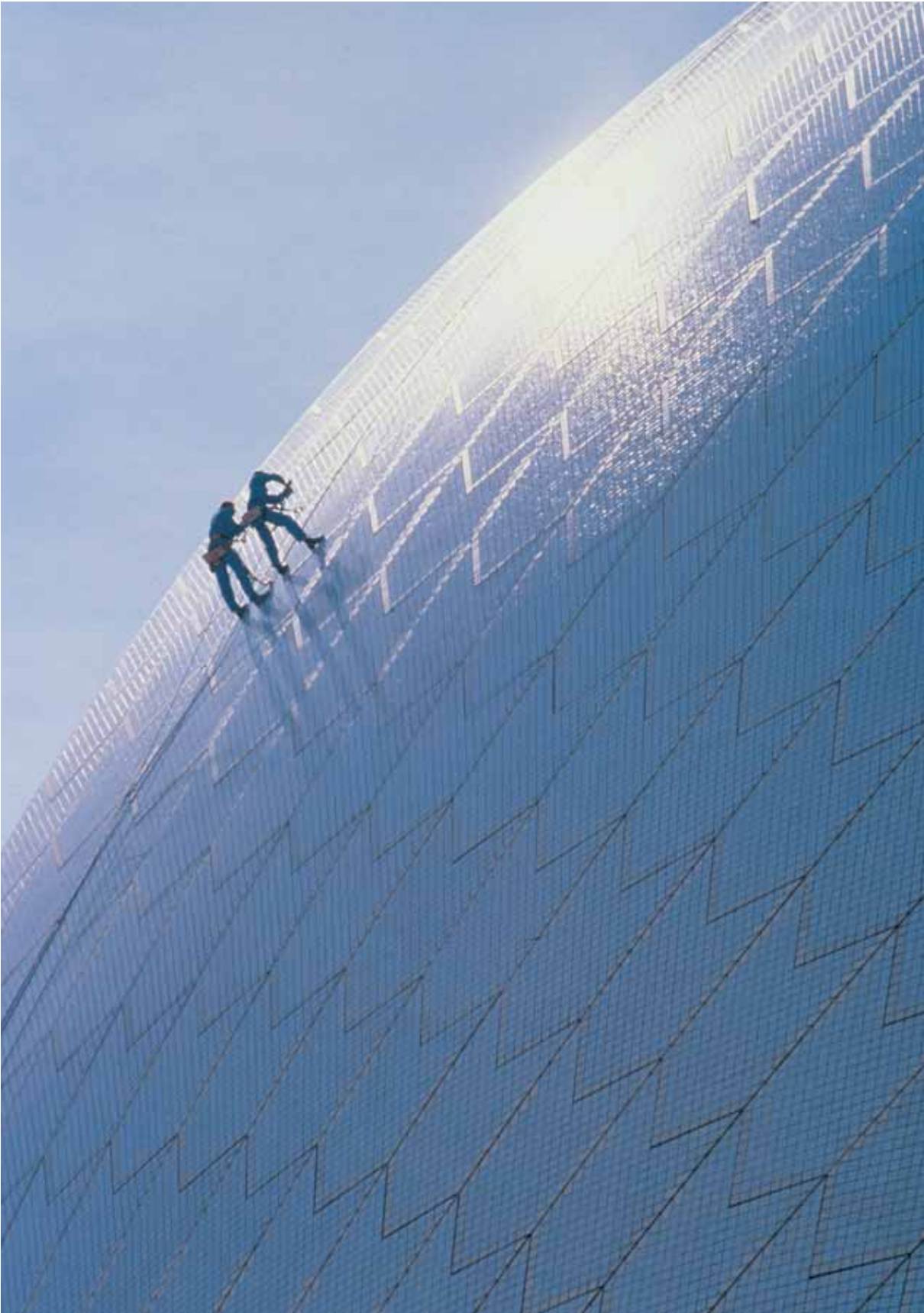
Figure 6.2 Monitoring the sealants to the tiling
