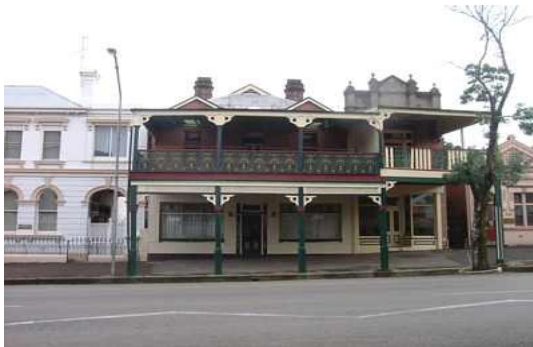
Restored verandah and shopfronts Photo courtesy of Comber Consultants Pty Ltd
