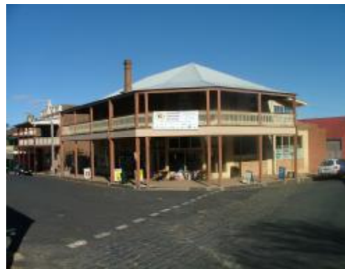
...and after the verandah reconstruction
