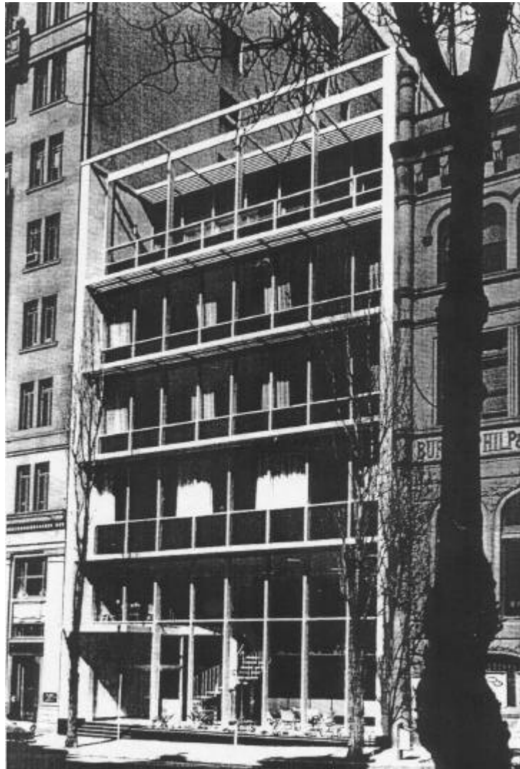
Figure 5: Liner House – Bridge Street Façade.
