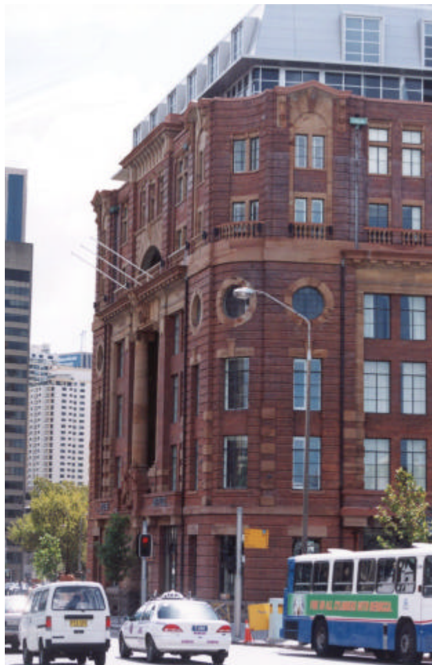
Figure 6: The former Parcels Post building, from Railway Square, Lee Street side.
