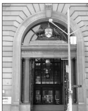
Major projects contributed to this year included the Walsh Bay development, Sydney Town Hall and the Westpac Bank in George Street. Photographs by Ed Beebe and Lianne Hall
