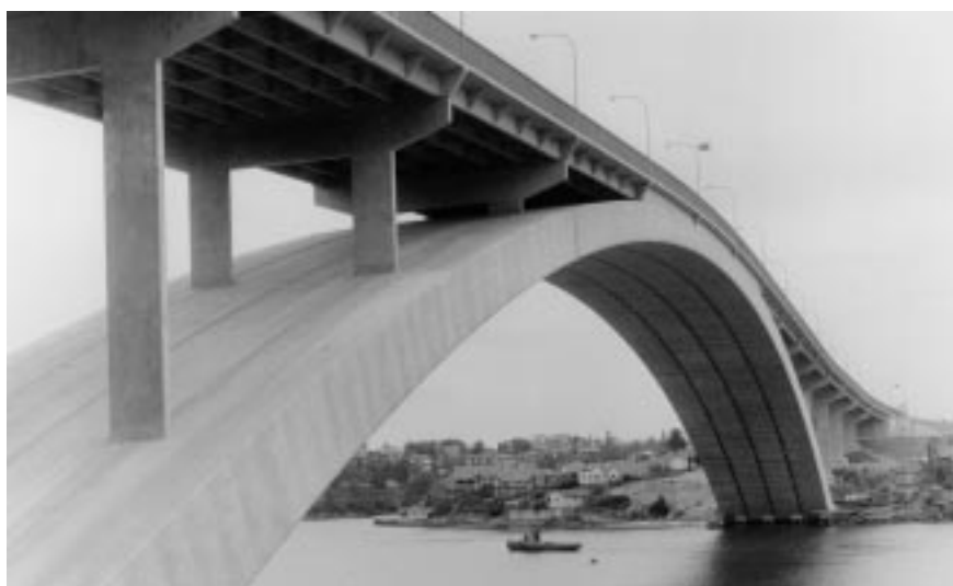
At the time of its opening in 1964, the Gladstone Bridge was the longest single-span concrete arch bridge in the world. This year the Heritage Council's Technical Advisory Group presented a technical seminar on conserving significant concrete structures of the 20th century. Photograph by Paul Percival, courtesy of the Australian Photograph Agency, State Library of NSW
