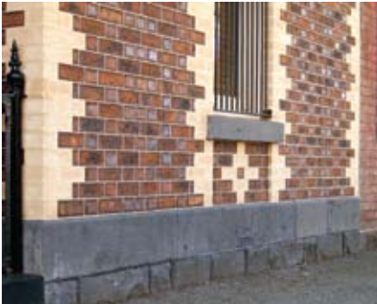
Figure 1 The dense bluestone base courses of this Melbourne building help reduce upward movement of moisture. Dense stones such as bluestones and granites are commonly seen as base courses around Australia.
