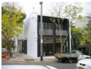
Council's Heritage Advisor provided advice on this infill development in Paddington, Architect Tina Engelen, for Woollahra City Council, New South Wales. Image courtesy Louise Thom, Woollahra City Council.
