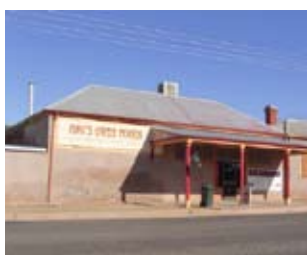
Frontage before and after verandah restoration. McDougall & Vines (2005) 'Broken Hill New South Wales - Verandah Program - 1998 - 2005 Summary Program'
