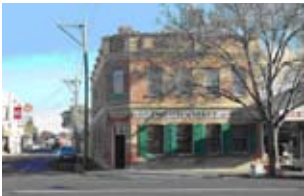
Former Haymarket Hotel prior to restoration, 1995 and following restoration, 2003. Images Ian Wynd and David Rowe.
