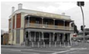
Maid & Magpie Hotel, South Australia, 1884 drawing and photo after restoration work, August 2008. Images and text courtesy Therese Willis, McDougall & Vines.
