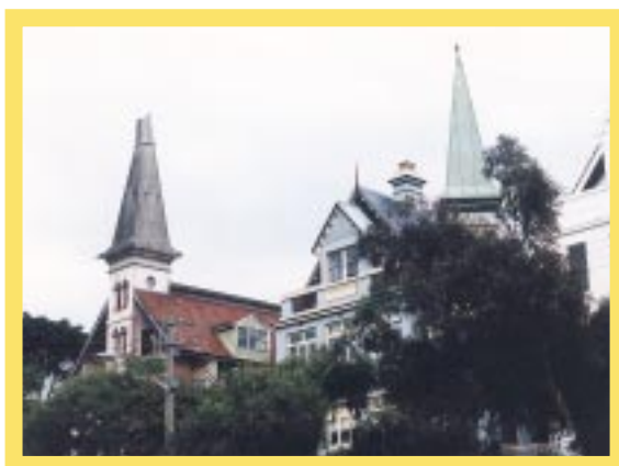
The houses forming the striking streetscape of 258-266 Johnston Street, Annandale, were built by well known Sydney builder John Young in the 1880s. Mass concrete was used in the footings and turrets.
