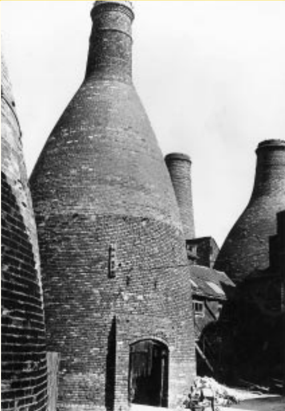
Bottle kilns similar to those used in cement production in the 19th century, photographed in 1889. Portland cement first began to be produced by Australian companies in the 1880s, including the Cullen Bullen Lime and Cement Company at Portland, NSW. Photograph courtesy of the Cement & Concrete Association of Australia
